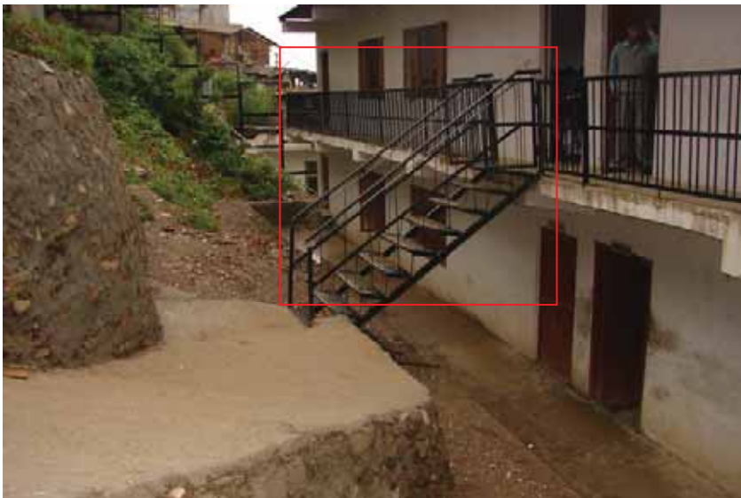
Providing additional staircase for easy evacuation
