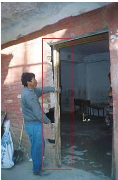
Changing doors - openings outwards for easy evacuation
