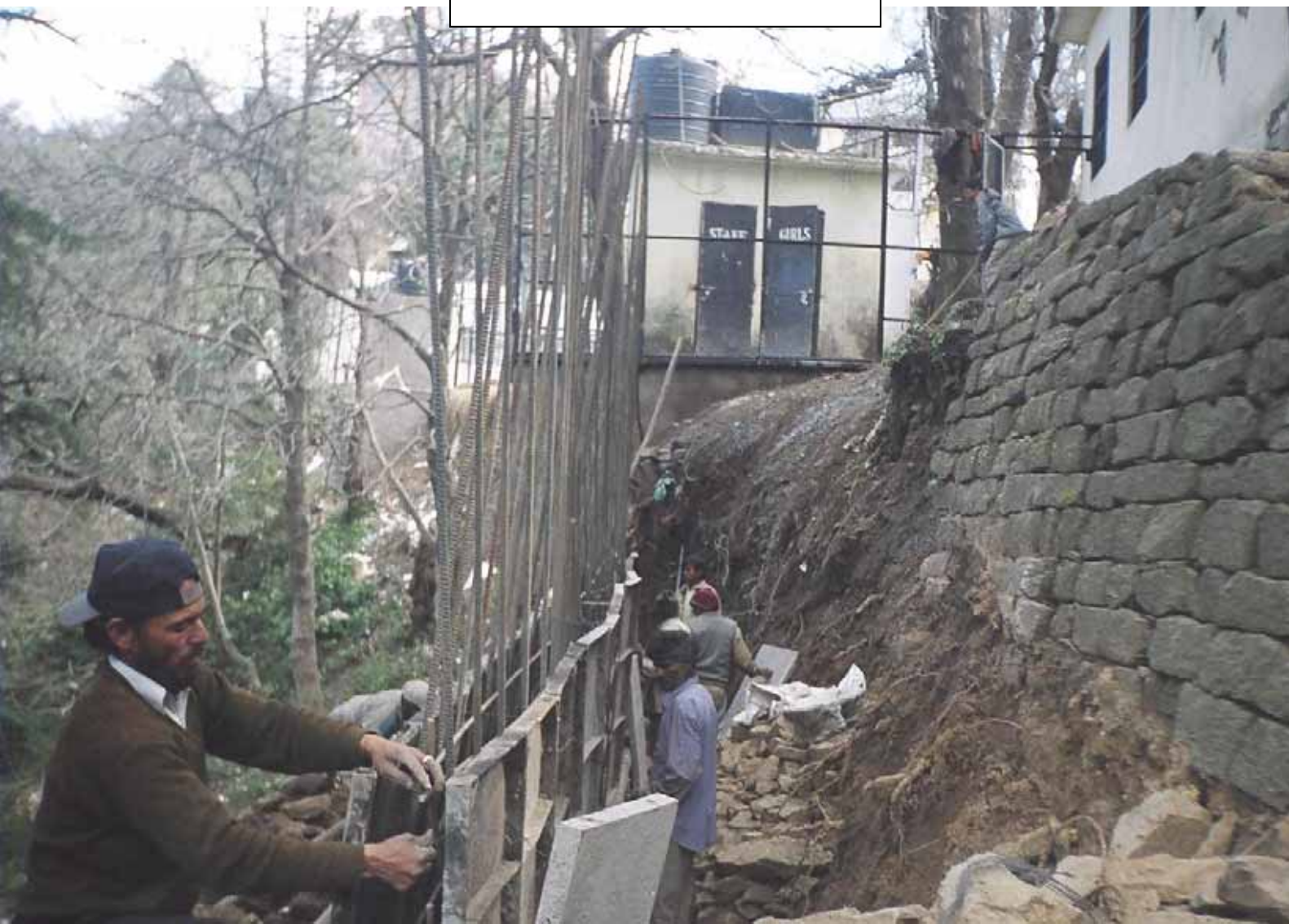
Construction of concrete retaining wall for slope protection
