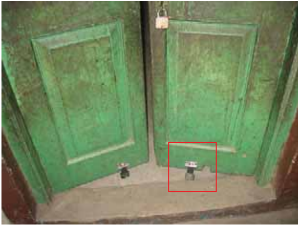
Providing stoppers on doors for easy evacuation
